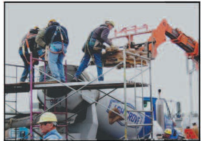
V-1 Grout mixed in a cement truck.
