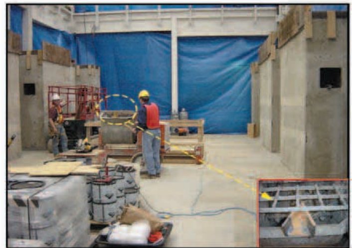
V-100 Epoxy Grout mixed in a paddle type power mixer with a two-bucket divider.
