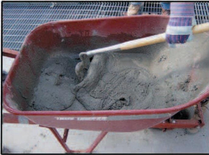
V-1 Grout mixed in a wheelbarrow with a hoe.
