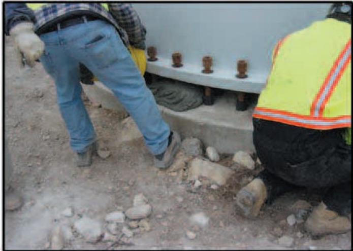
Placing V-1 Grout for large equipment ring.
