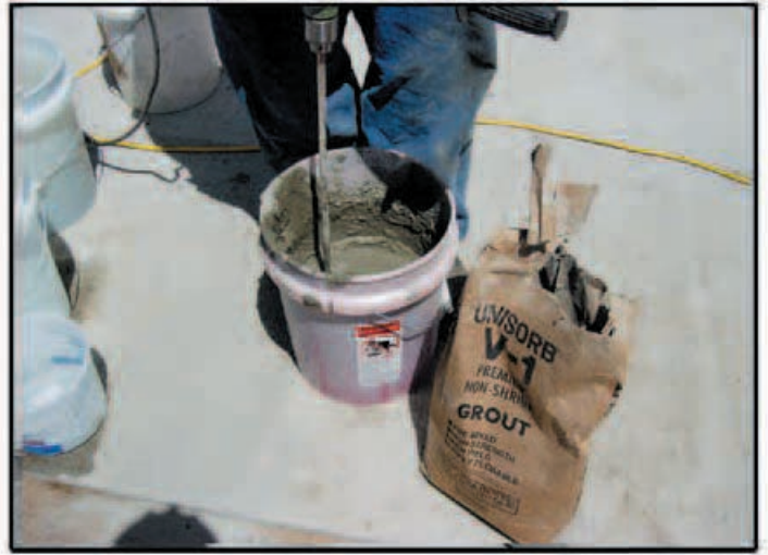
V-1 Grout mixed in a pail with a power drill and paddle.
