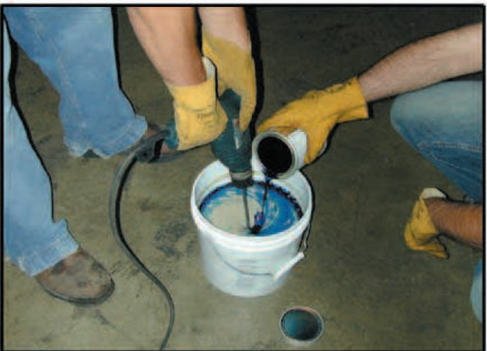
Standard V-100 Epoxy Grout mixed in a pail with a power drill and paddle.
